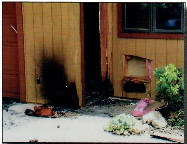
These images from a Gila County Cooperative Extension webinar available online show some of the ways embers from a distant wildfire can claim a home – including unscreened vents and debris against a wall (top), flammable material on a porch (below) and flower beds and window flower boxes against the house (bottom).
